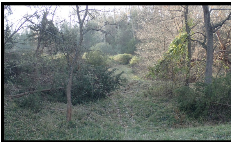
This photo is of a EQIP project currently in progress. The landowner is removing cedar trees off his site in the Loess Hills.
